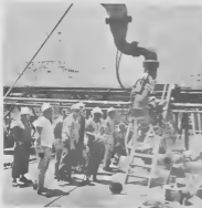
Oil Movts. Shift Foreman Julian Daniel (Picture left & right) shows how to operate control box to hook up metal loading arms. In center is a hydraulic coupling device to connect on tanker flange.
